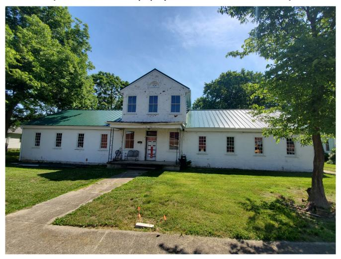
After the flooring, we tore out the old windows and bought \$24,000 of new Anderson windows. We were able to replicate the rare "9 over 6" original windows in the front of the building, preserving a unique look. After the windows were installed, exterior trim was contracted locally at a cost of roughly \$2,500.00 (thanks to a matching donation from Miller Lumber).
